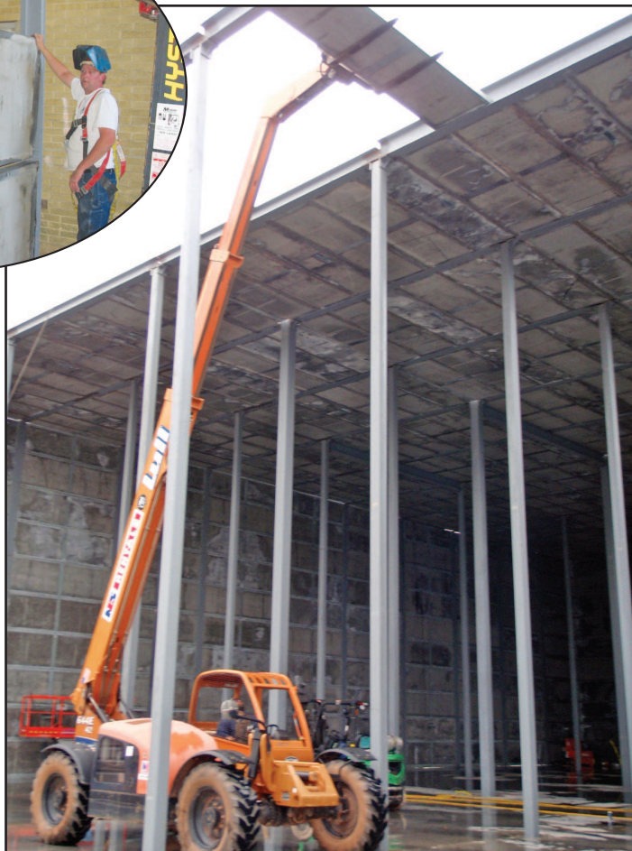
Fig. 2. Custom Vault's panels form both the walls (left) and the roof of a very large pharma vault
